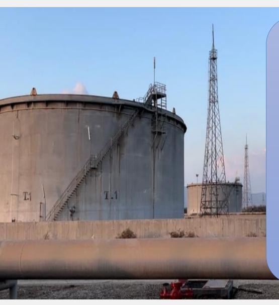
Three floating roof Tanks with 11,300 cube meter capacity
